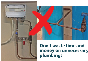
Remote sensors eliminate need for bypasses
