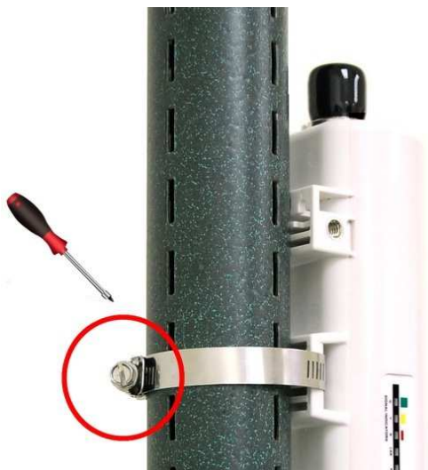
Figure 9 Pole Mounting – Step 2
