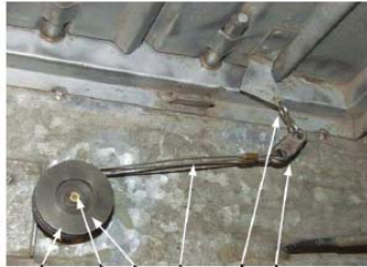
Wrap spring clutch break Remove and discard old clutch break, shaft, cable, fusible link, and hook.
